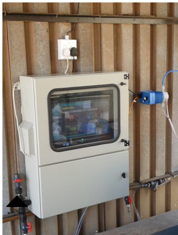
RAPID installation in South Africa
